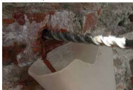
Abb. 5 Pfeiler 18, TP2, 'flüssige' Probe!!
