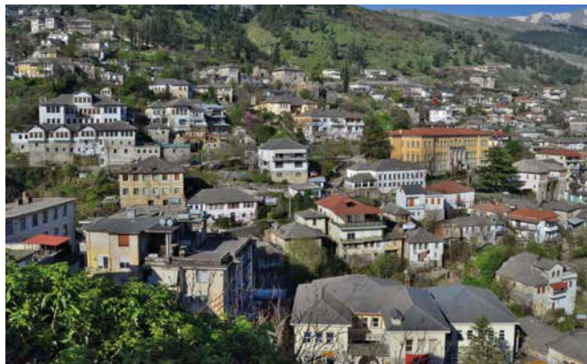
Fig. 6: View of Palorto Quarter, Gjirokastra. The Ottoman character of this residential area has almost been lost due to new constructions, red tile roofing and modern additions.
