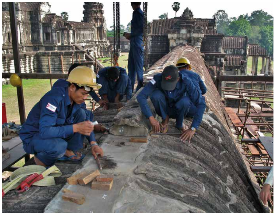
Fig. 2: Roof conservation on the Churning of the Sea of Milk Gallery, 2009
