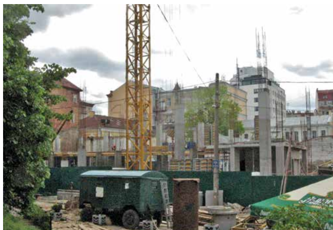
Fig. 3: Construction of a new building that has begun at 3-5 Desyatynny Lane.
