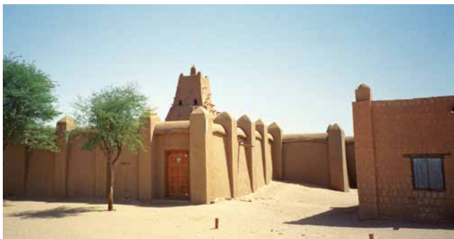
Fig. 1: The Sankoré Mosque in Timbuktu, a UNESCO World Heritage site, was severely damaged by the jihadists, but has been restored since then. Photo: wikipedia
