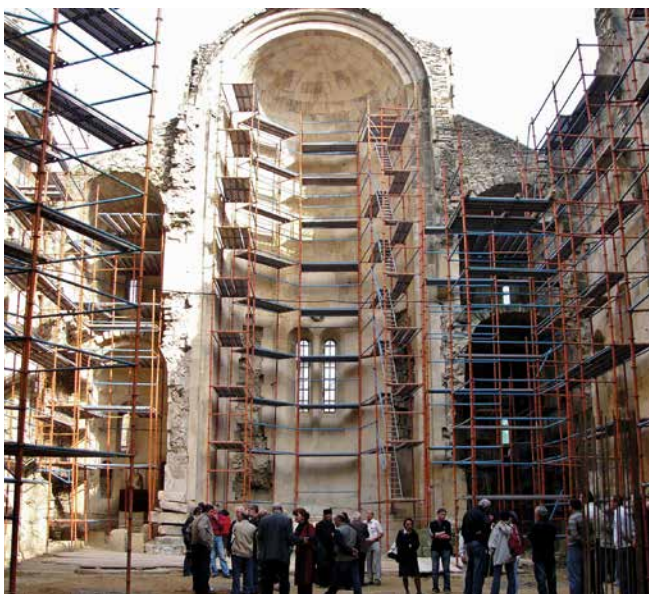
Fig. 2: October 2009. A team of experts and officials inspecting the reconstruction works on Bagrati Cathedral after they had been stopped as a result of public campaign. Photo: ICOMOS Georgia
