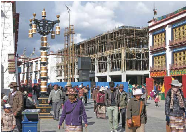
Fig. 5: The Tsona Tsongkhapa house, under construction in 2013. In spite of the close proximity to the Jokhang temple, a UNESCO site, and the efforts to preserve the historic buildings, the approach to conserve the historic houses is still the replacement of historic buildings by new constructions. Photo: Ken Okuma / Tibet Heritage Fund
