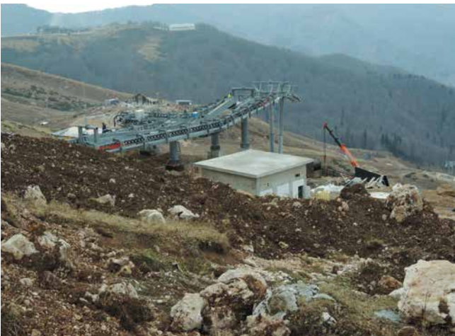
Fig. 2: Construction of the cable cars to the ski resort.
