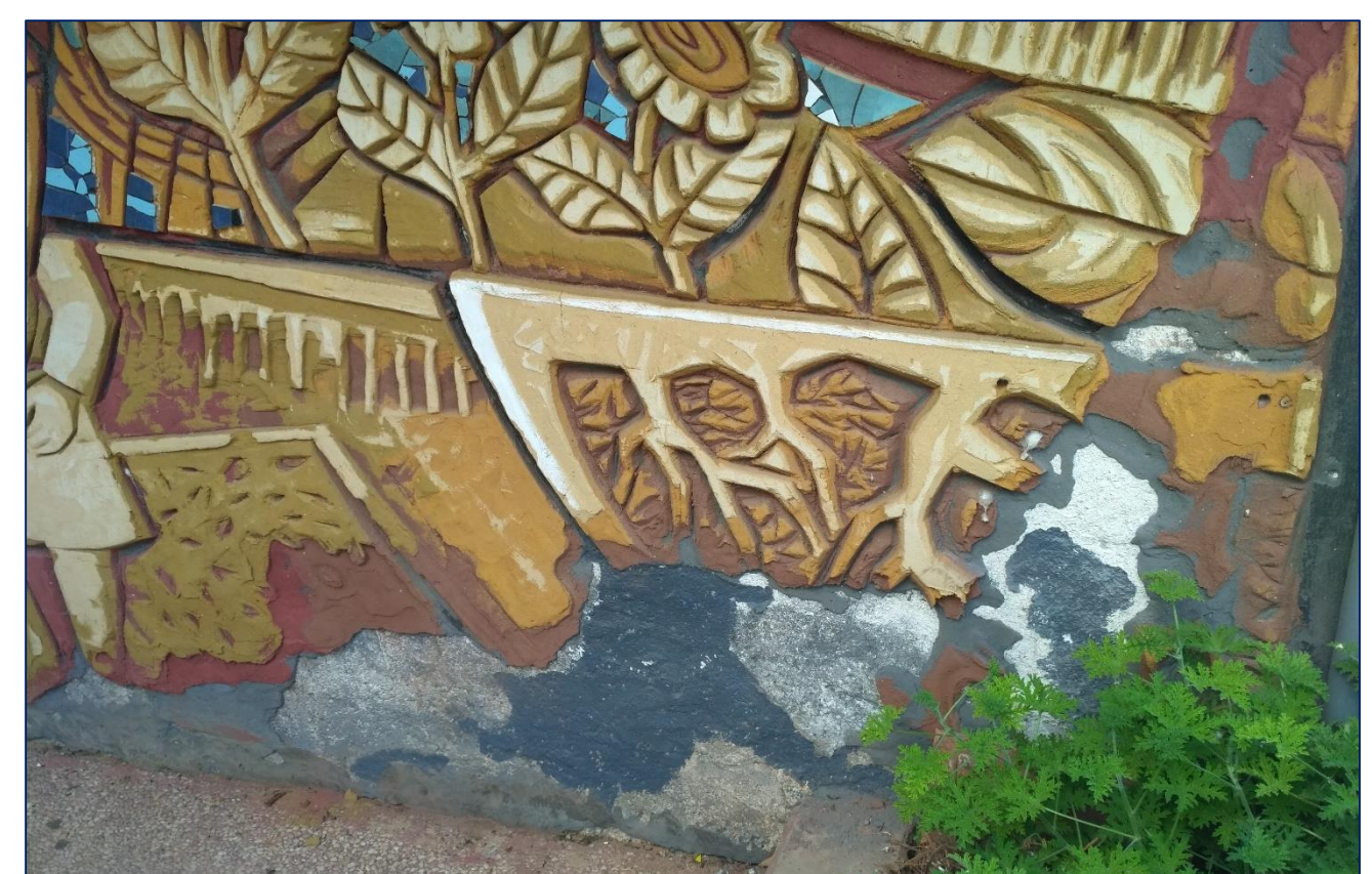
Crambling and separation because of capillary action
