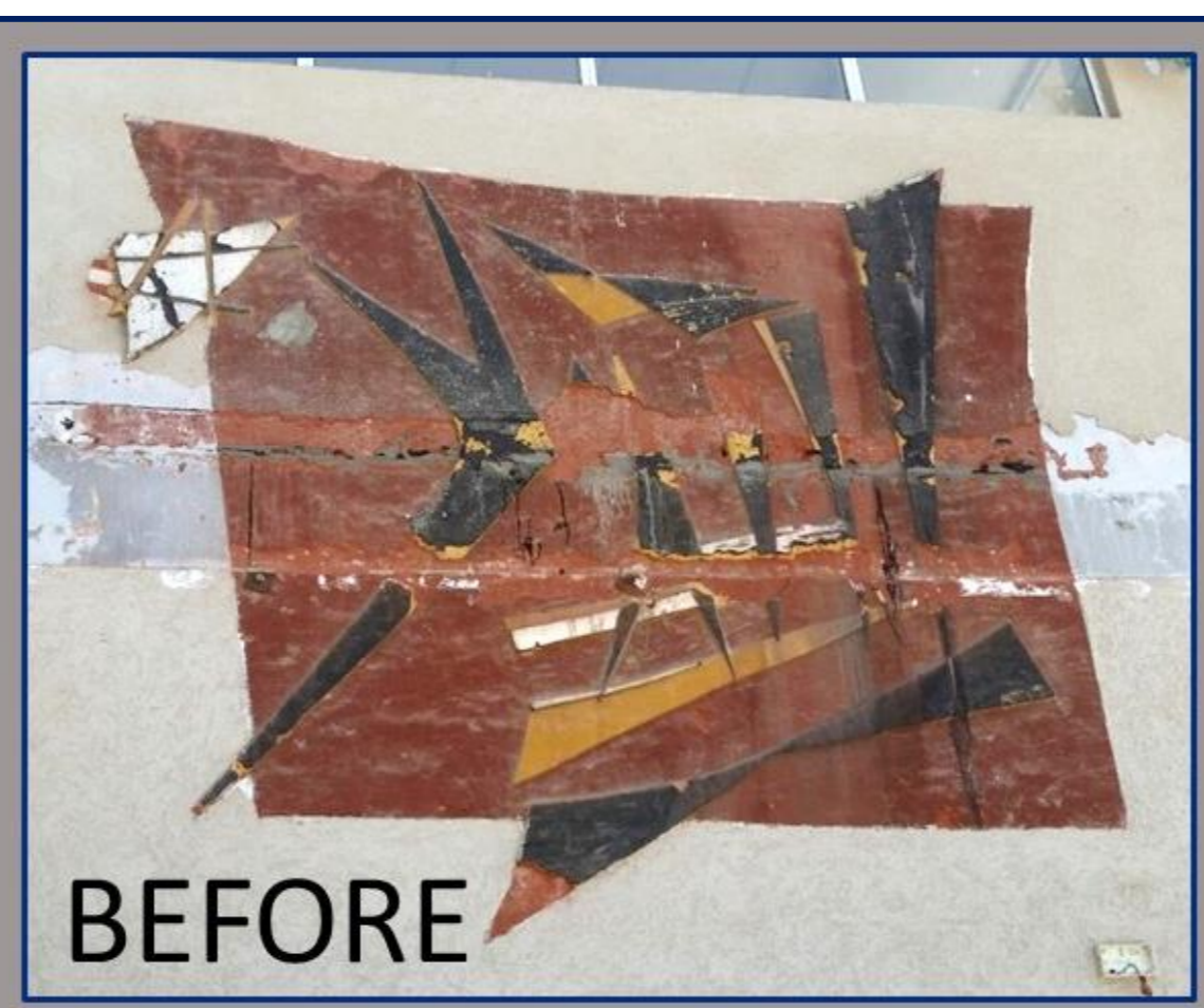
Laden injection between loose parts of Sgraffito
