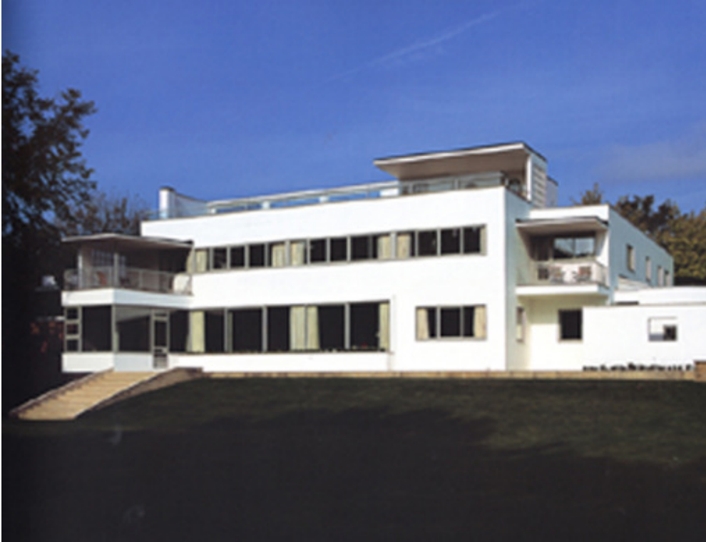
Fig. 3 Miramonte – As restored, 2003
