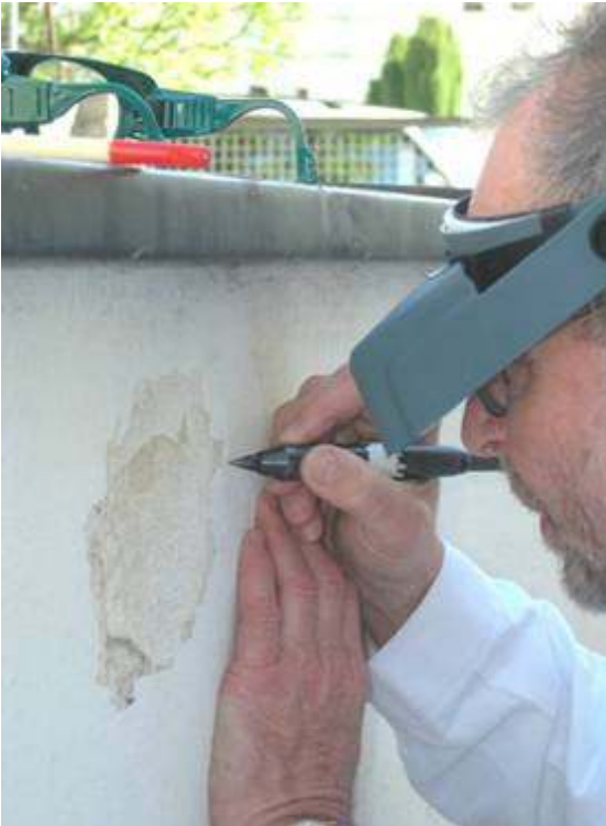
(7) Brno, Tugendhat House, 1828-30, Ludwig Mies van der Rohe, northwest façade, parapet, southeast side, May 2004: First tests using pneumatic scissile to a careful detachment of the harmful coating consisting of cement grout and paint with artificial resin dating from 1985. Photo: HAWK/Hitzler
