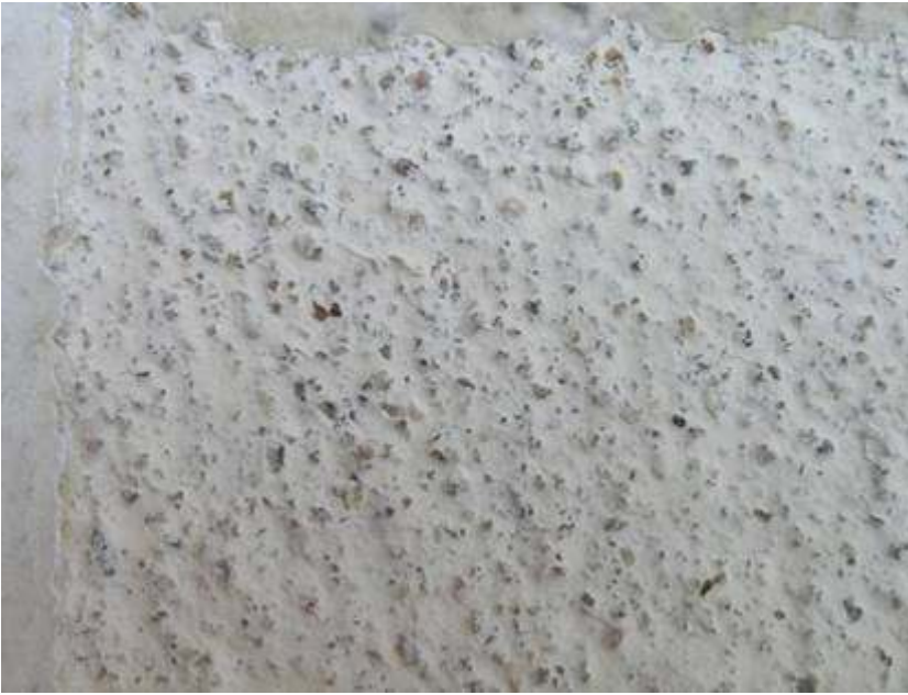
(6) Brno, Tugendhat House, 1928-30, Ludwig Mies van der Rohe, southwest façade, upper terrace, wall of boys sleeping room, detail, after cleaning 2004. The surface appears in a stone like colour. The rendering consisting of hydraulic lime mortar is smoothed with a wooden board. The yellowish lime paint is applied in such a manner, that the grains of the sand in the mortar appeared at the surface and were part of the polychrome. The thin paint contributed to the refining of the materiality of the surface.
