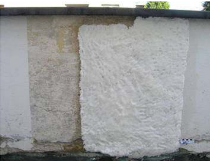
(8) Brno, Tugendhat House, 1828-30, Ludwig Mies van der Rohe, northwest façade, parapet, southeast side, May 2004: Chemical conversion of the sulphated original surface of the rendering and compresses to diminish the soluble salts concentrated at the surface. Photo: HAW / Hammer.
