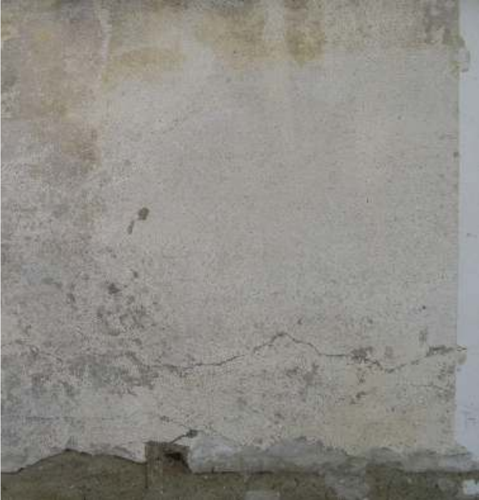
(9) Brno, Tugendhat House, 1828-30, Ludwig Mies van der Rohe, northwest façade, parapet, southeast side, May 2004: Effect of chemical cleaning. After the conversion of the gypsum the appearance of the surface is much brighter, but not white. Photo: HAWK/Hammer
