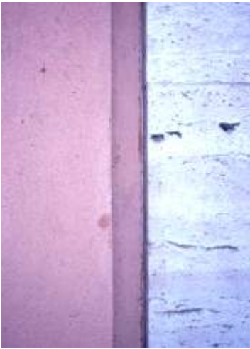
(4) Potsdam, Neubabelsberg, Urbig House 1915-17, Mies van der Rohe. The rendering of the facade has been renewed after detachment of the original one 1990. the difference between copy and original is no longer perceptible. Photo Hammer 2001.
