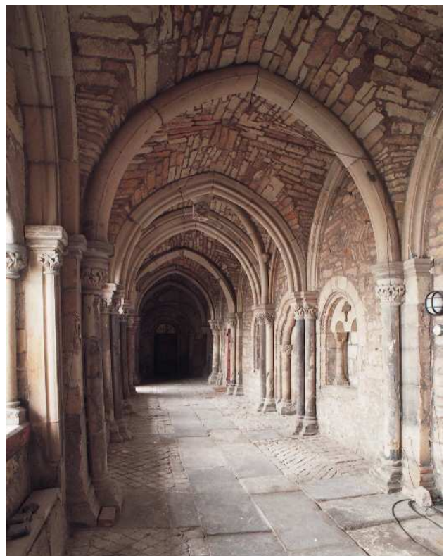
Fig.1 Cloister of St.Michael's Church, west wing
