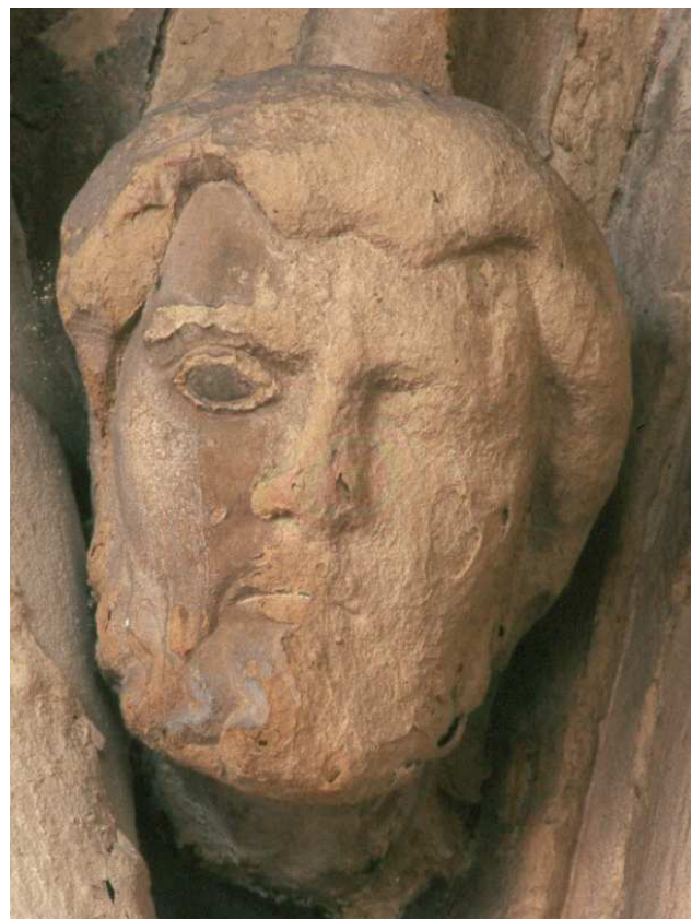
Fig.2 Cloister of St.Michael's Church, vault springer, showing stone deterioration
