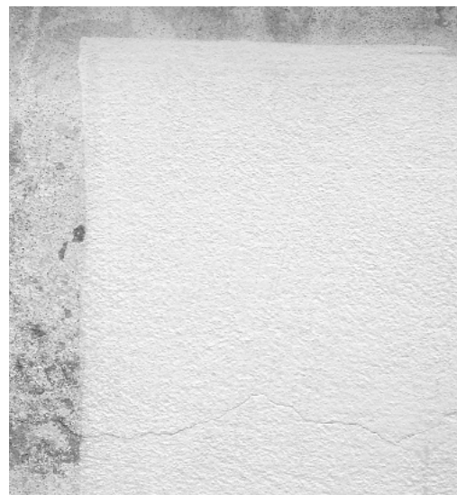
Brno, Tugendhat House, 1828-1830, Ludwig Mies van der Rohe, northwest facade, parapet, southeast side, May 2004: First test of a thin lime wash coloured with fine suspension of local sand. This coloured lime wash takes over the original technique of surface coating and may be seen not only as protection of the original surface but also as a technique of sustainable maintenance. Photo HAWK, Ivo Hammer.
