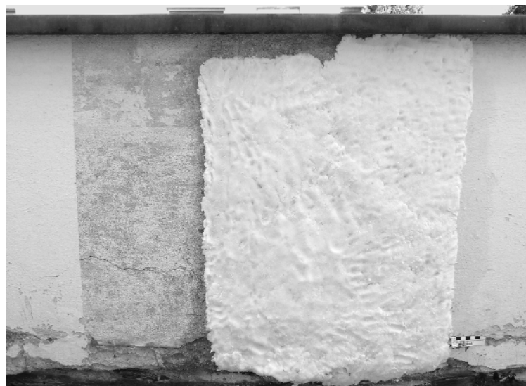
Brno, Tugendhat House, 1928-30, Ludwig Mies van der Rohe, northwest facade, parapet, southeast side, May 2004: Chemical conversion of the sulphated original surface of the rendering and compresses to diminish the soluble salts concentrated at the surface. Photo HAWK, Ivo Hammer.
