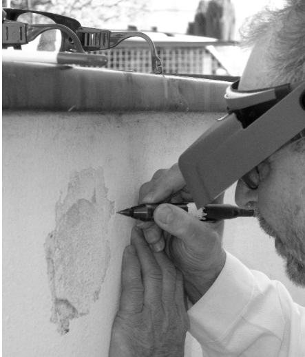
Brno, Tugendhat House, 1828-30, Ludwig Mies van der Rohe, northwest facade, parapet, south-east side, May 2004: First tests using pneumatic scissile to a careful detachment of the harmful coating consisting of cement grout and paint with artificial resin dating from 1985. Photo HAWK, Christine Hitzler.
