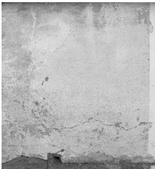
Brno, Tugendhat House, 1828-30, Ludwig Mies van der Rohe, northwest facade, parapet, southeast side, May 2004: Effect of chemical cleaning. After the conversion of the gypsum the appearance of the surface is much brighter, but not white. Photo HAWK, Ivo Hammer.
