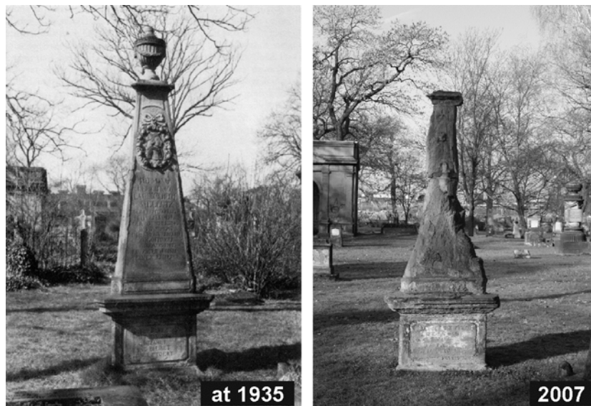
Figure 1: Historical and present-day photo showing the condition of the Sielentz obelisk exhibits strong weathering and a loss of ornamental designs.
