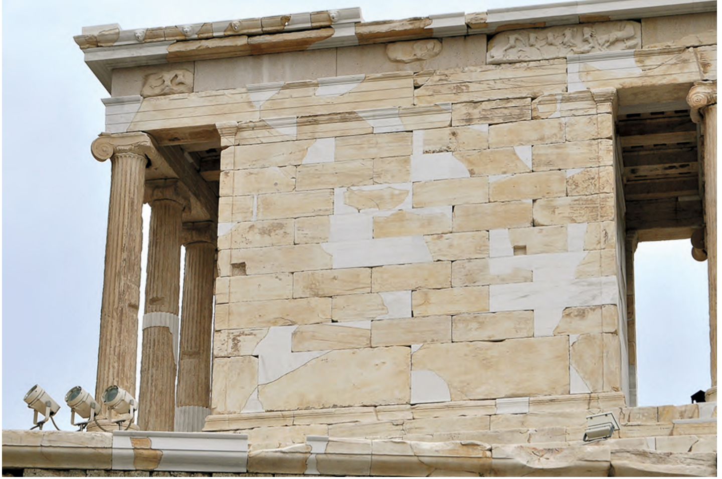
Marble inserts in the façade of the Erechtheion of the Acropolis, Athens (Greece), 421 and 406 BC; Photo: 2014, UPV (Pilar Bosch)
