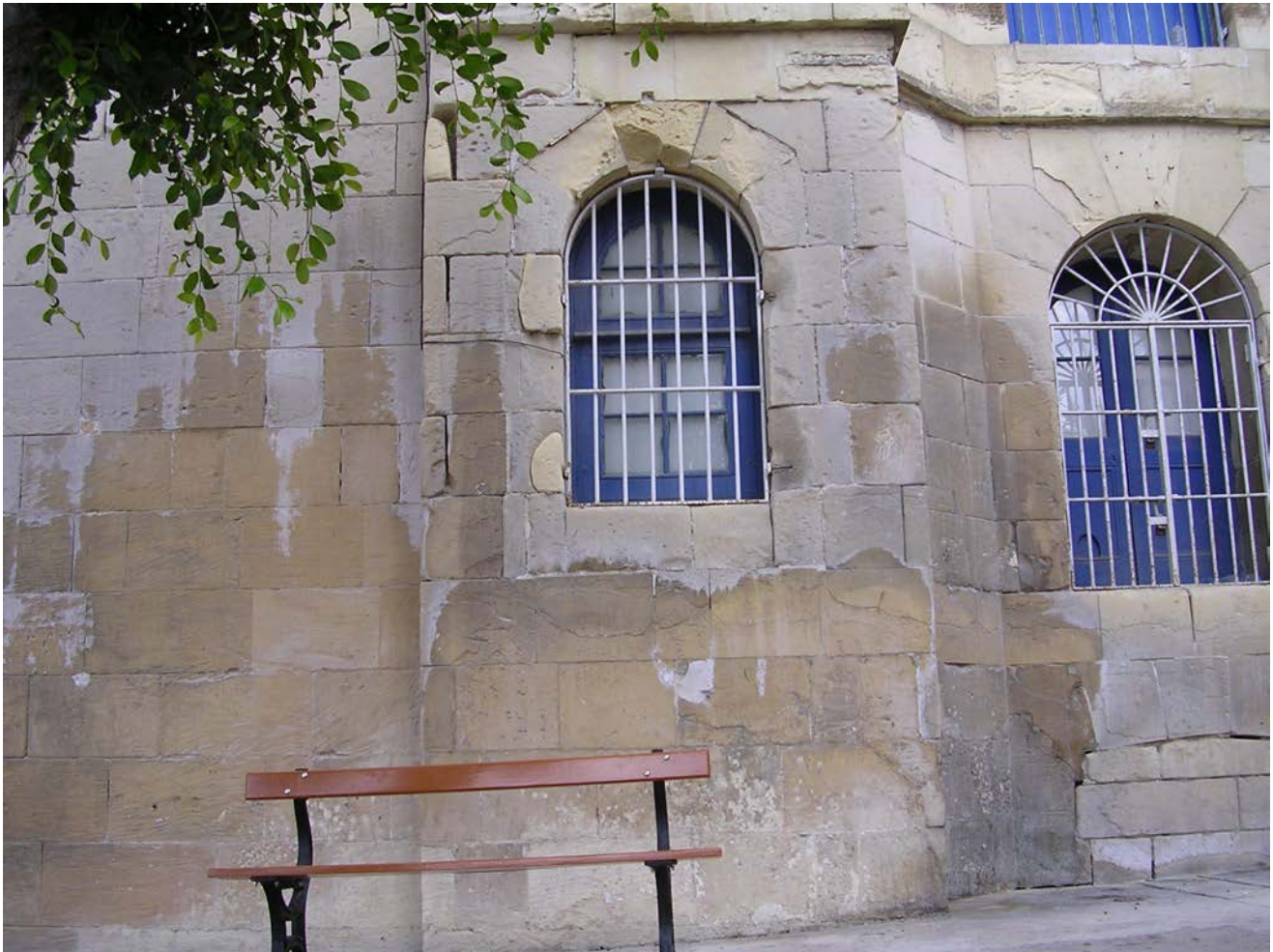
Hygroscopic salts have resulted in a damp patch on a limestone wall (Malta); Photo: 2008, UM (JoAnn Cassar)
