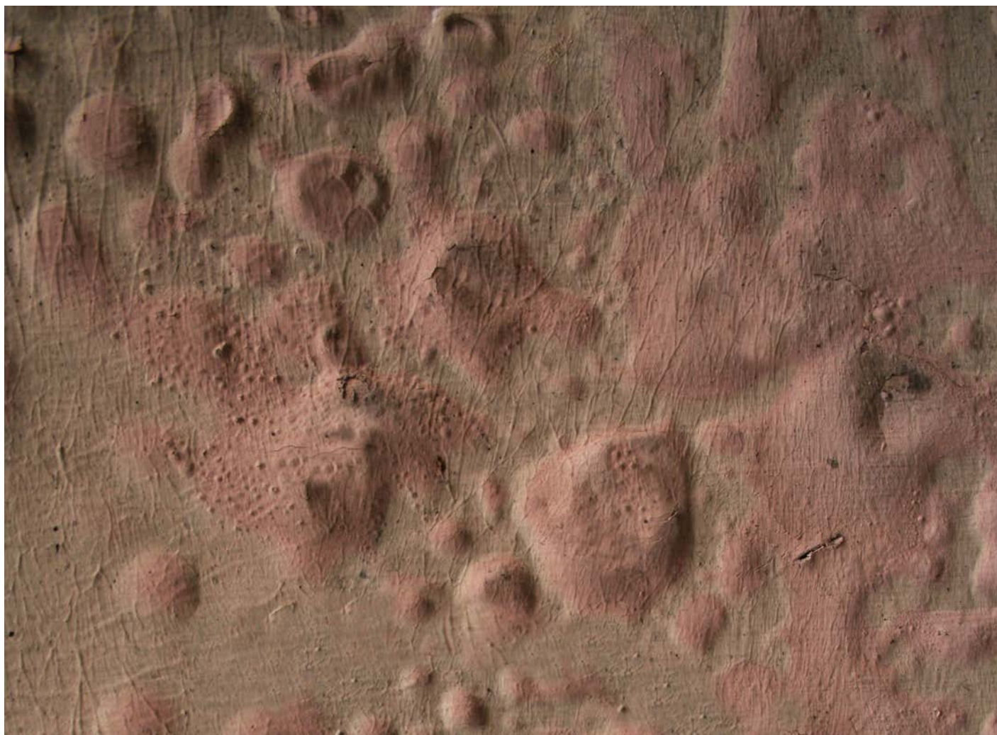
Paint layers showing bulges, Secco wall painting, Cluj-Napoca (Romania), 19th century; Photo: 2015, UAD (Adrian Rauca)
