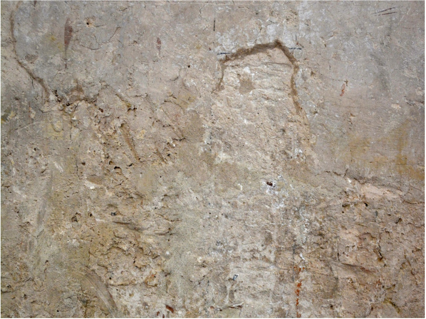
Coarse layer of arriccio (lower section) under intonaco, Chapel of St. Helen, Šenkovec (Croatia), late 14th century; Photo: 2014, HRZ (Katarina Gavrilica)
