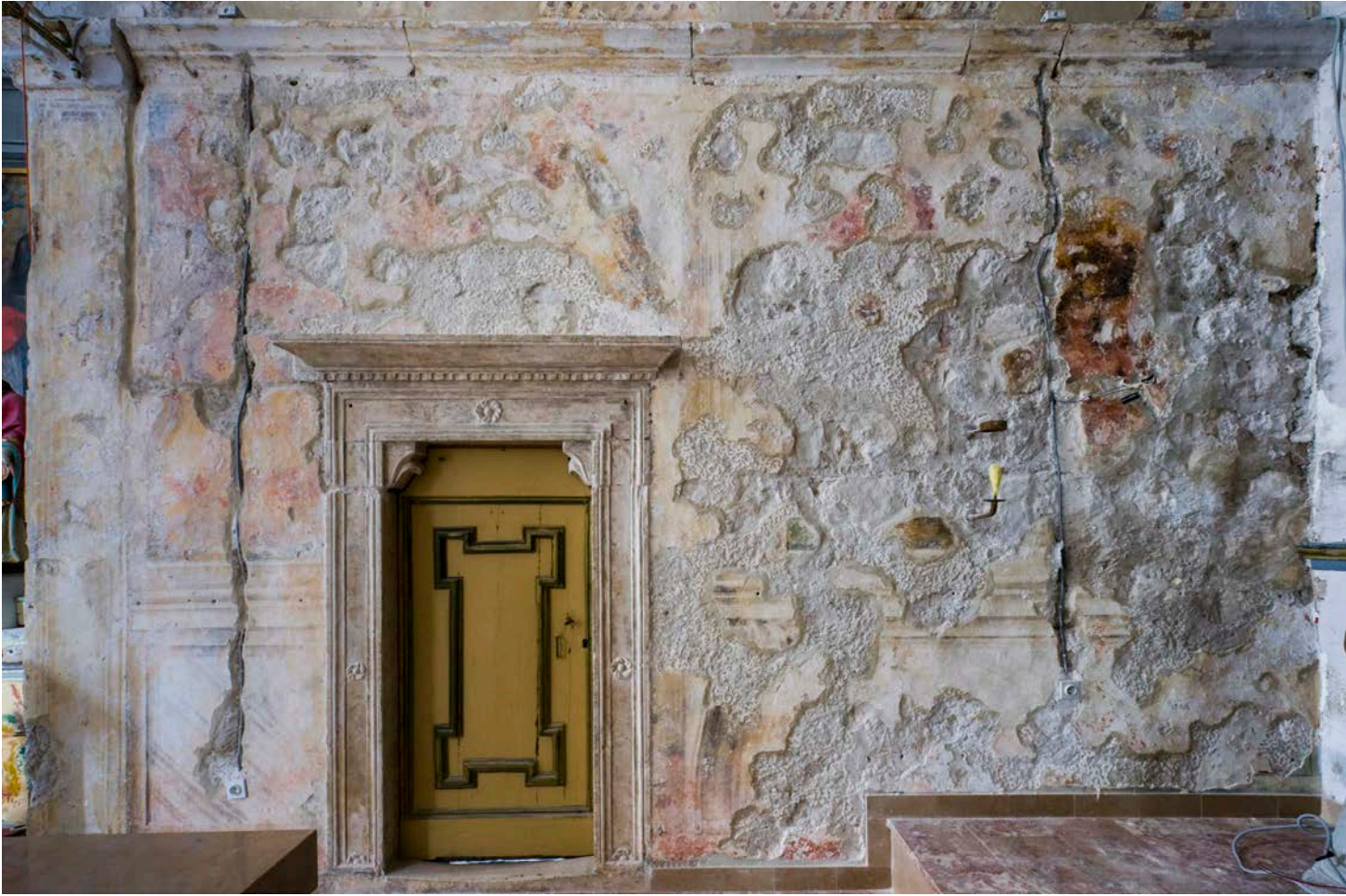
Mortar additions along the borders of historic plaster, Church of St. Vitus, Modestus and Crescentia, Trsteno (Croatia), 16/17th century; Photo: 2010, HRZ (Katarina Gavrilica)
