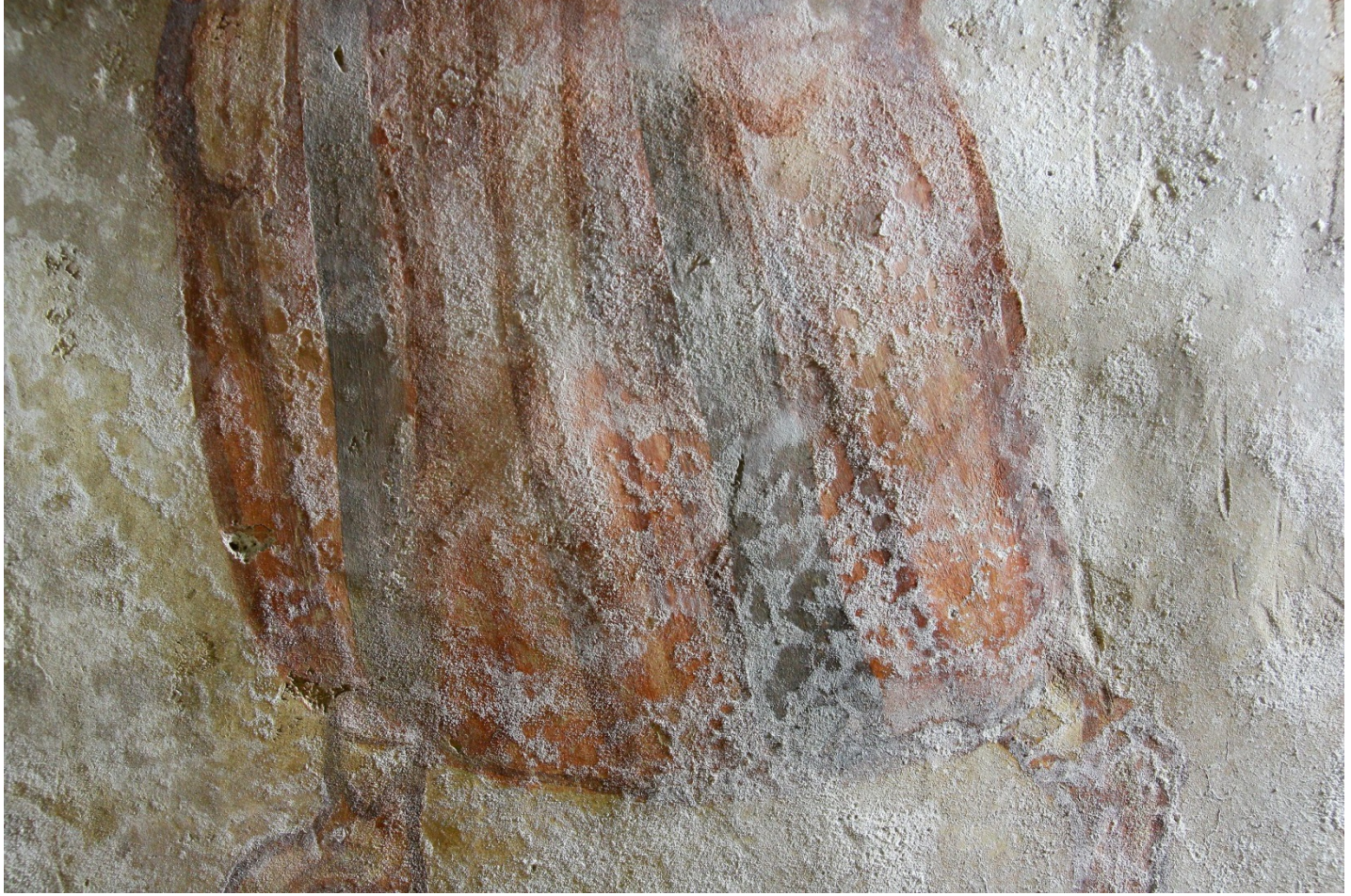
White salt efflorescence, Roman tomb, Siliistra (Bulgaria), 4th century AD; Photo: 2014 (Stefan Belishki)
