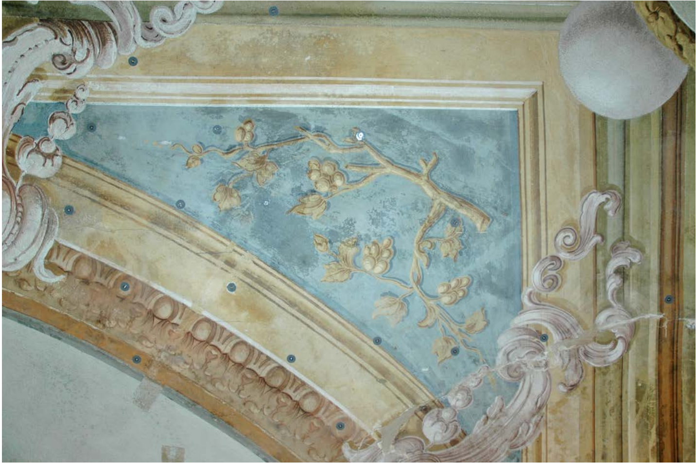
Painting on a ceiling secured by screws, Sorkočević Palace (Bishop's Palace), Dubrovnik (Croatia), 18th century; Photo: 2008, HRZ (Ivan Srša)
