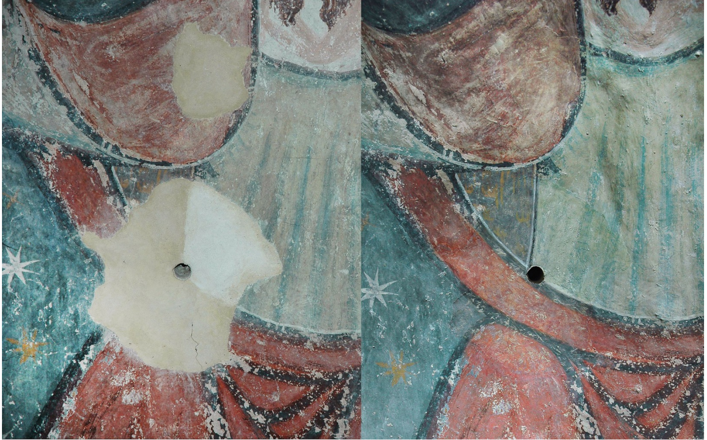
Before/after mimetic reintegration of an infill, Church of St. Lawrence, Požega (Croatia), 12th century; Photos: 2012, HRZ (Ivan Srša)
