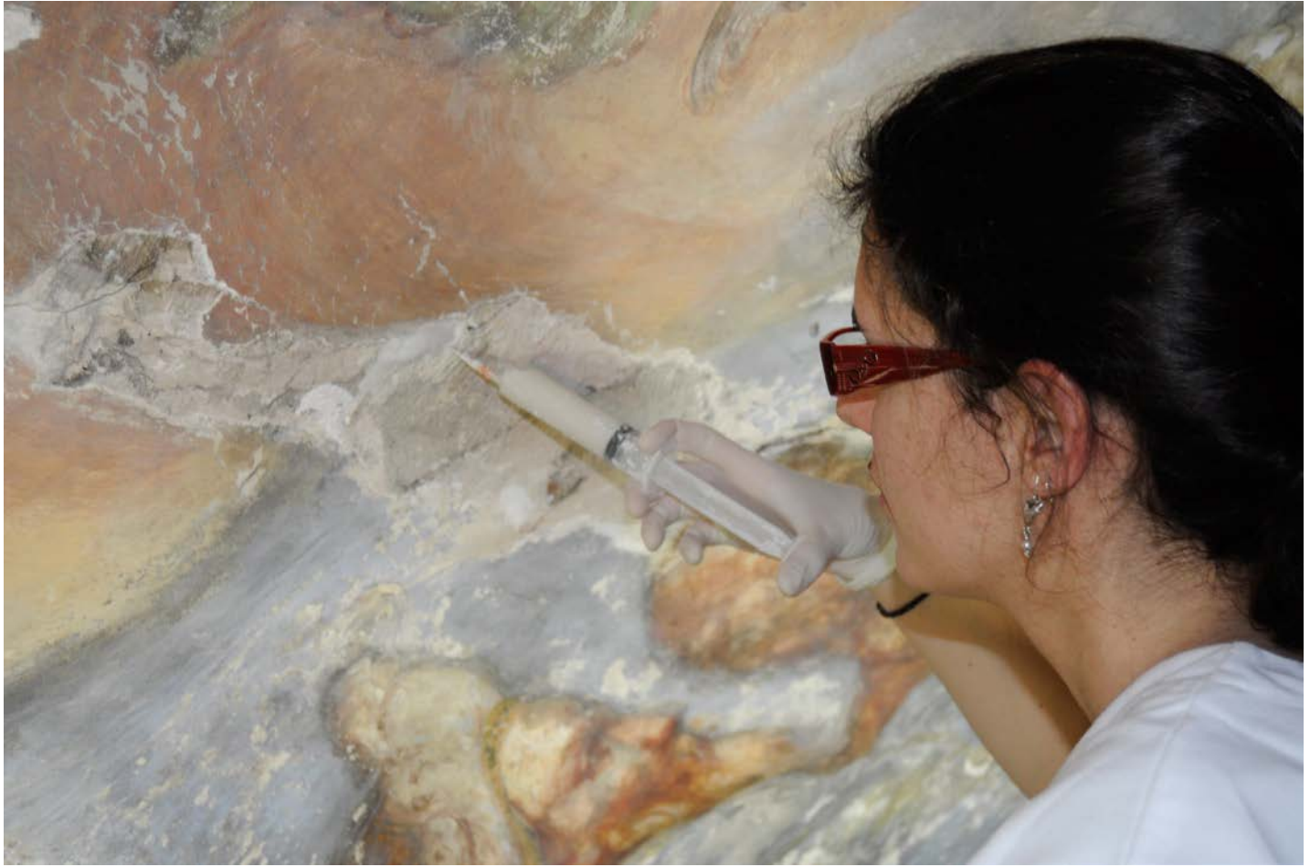
Injection of a grout, wall painting by Dionis Vidal, Church of San Nicolás Obispo y San Pedro Mártir, Valencia (Spain), 1694-1700; Photo: 2014, UPV
