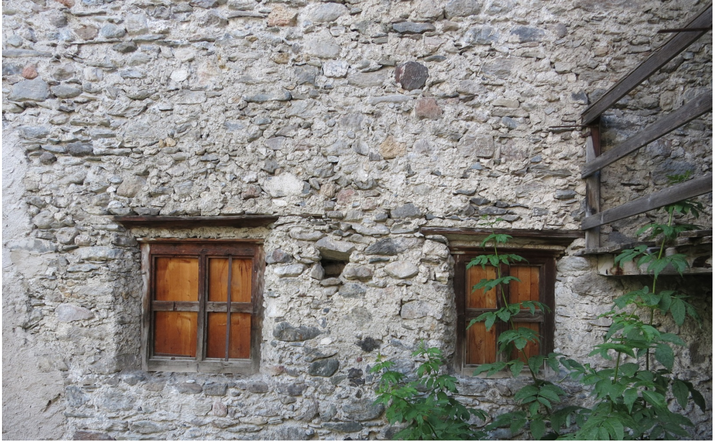
Typical rubble masonry, historic building, Santa Maria Val Müstair (Switzerland); Photo: 2015, HAWK (Angela Weyer)
