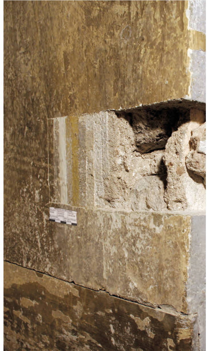
Areas of uncovering, showing successive superimposed paint layers, in a show flat, La Cité Radieuse by Le Corbusier, Marseille (France), 1952 (left); similar uncovering of layers of paint and plaster for an investigation, Church of Saint Nicholas, Ribița (Romania), 15th century (right); Photos: 2015, CICRP (Odile Guillon), 2014, UAD (Adrian Rauca)
