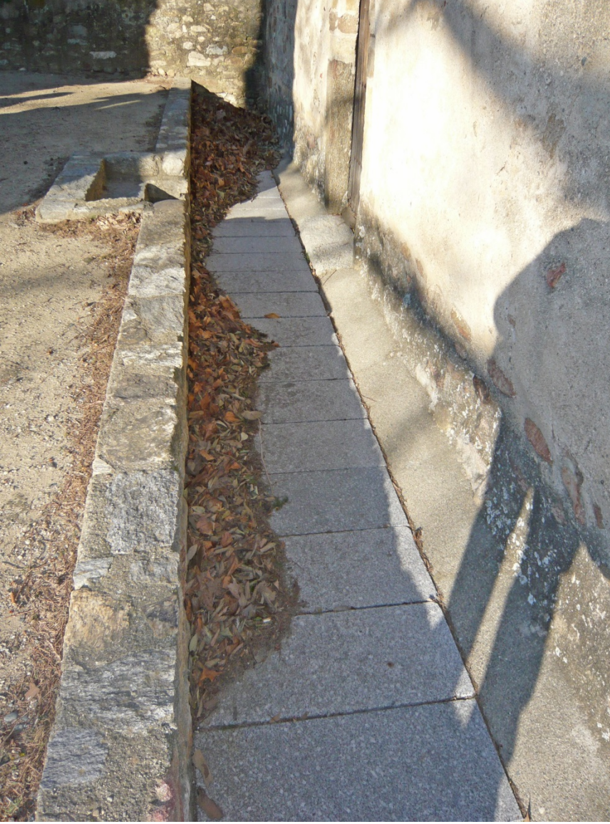
Channel around the Chapel of Saint Martin de Fenollar, Maureillas-las-Illas (France), 12th century; Photo: 2012, CICRP (Jean-Marc Vallet)
