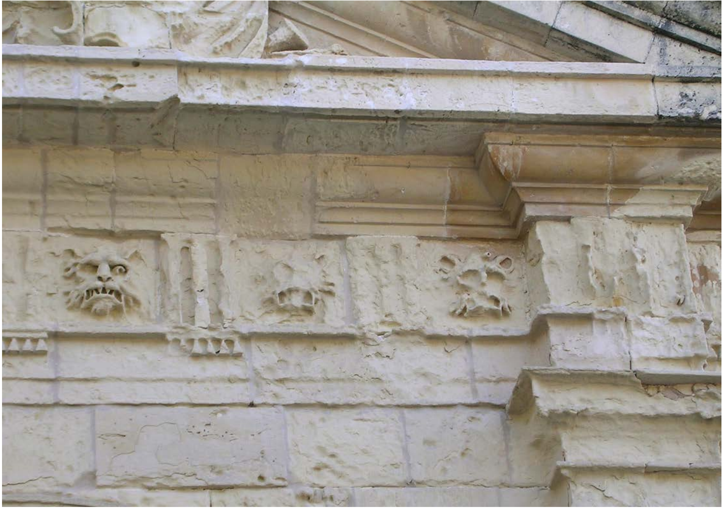
Fluctuating environmental conditions, especially humidity, have led to the deterioration of this salt-laden limestone (part of upper frieze in Globigerina Limestone), Greek's Gate, Mdina (Malta), early 18th century; Photo: 2008, UM (JoAnn Cassar)
