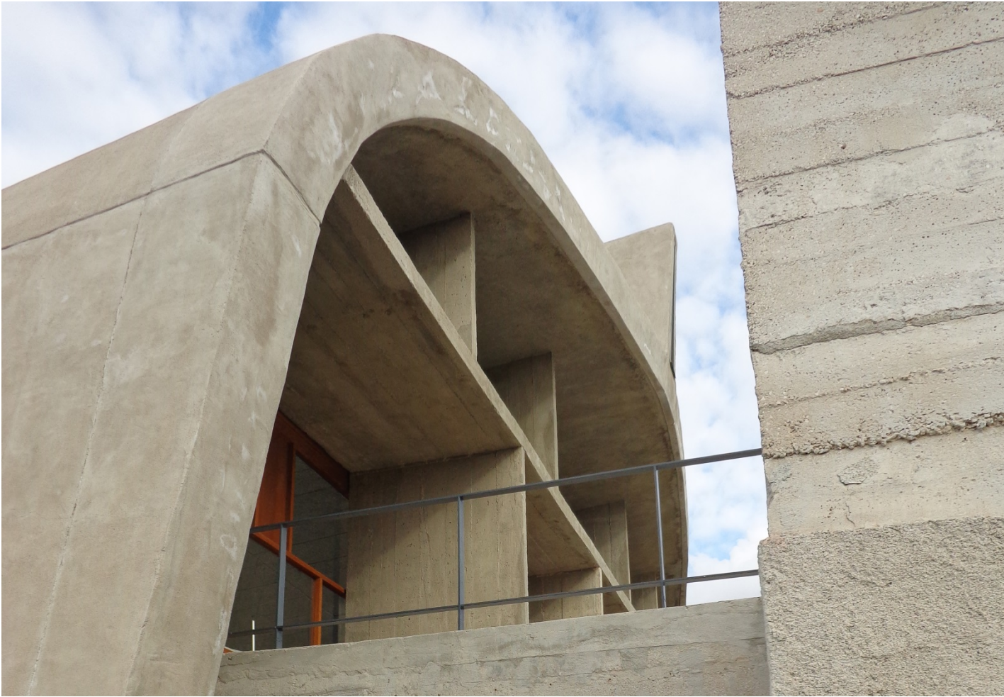
Different concrete surface finishes, La Cité Radieuse by Le Corbusier, Marseille (France), 1952; Photo: 2015, RPS (Dörthe Jakobs)
