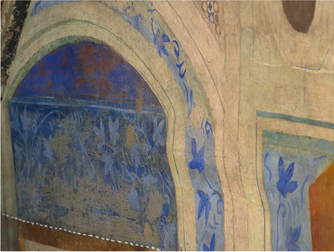
Convex deformation of painted plaster layer, Chapel of Saint-Martial, Palais des Papes, Avignon (France), 14th century; Photo: 2013, CICRP (Jean-Marc Vallet)
