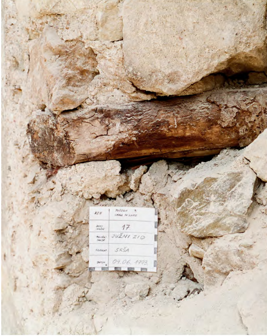
Remains of a wooden cross-bar in a putlog hole (left), Church of St. Lawrence, Požega (Croatia), late 13. century; Photo: 1993, HRZ (Ivan Srša); open putlog holes in a wall (top right) and detail (bottom right), Church of The Blessed Virgin of the Rosary, Remetinec (near Novi Marof), second half of 15th century; Photo: 1992, HRZ (Ivan Srša)
