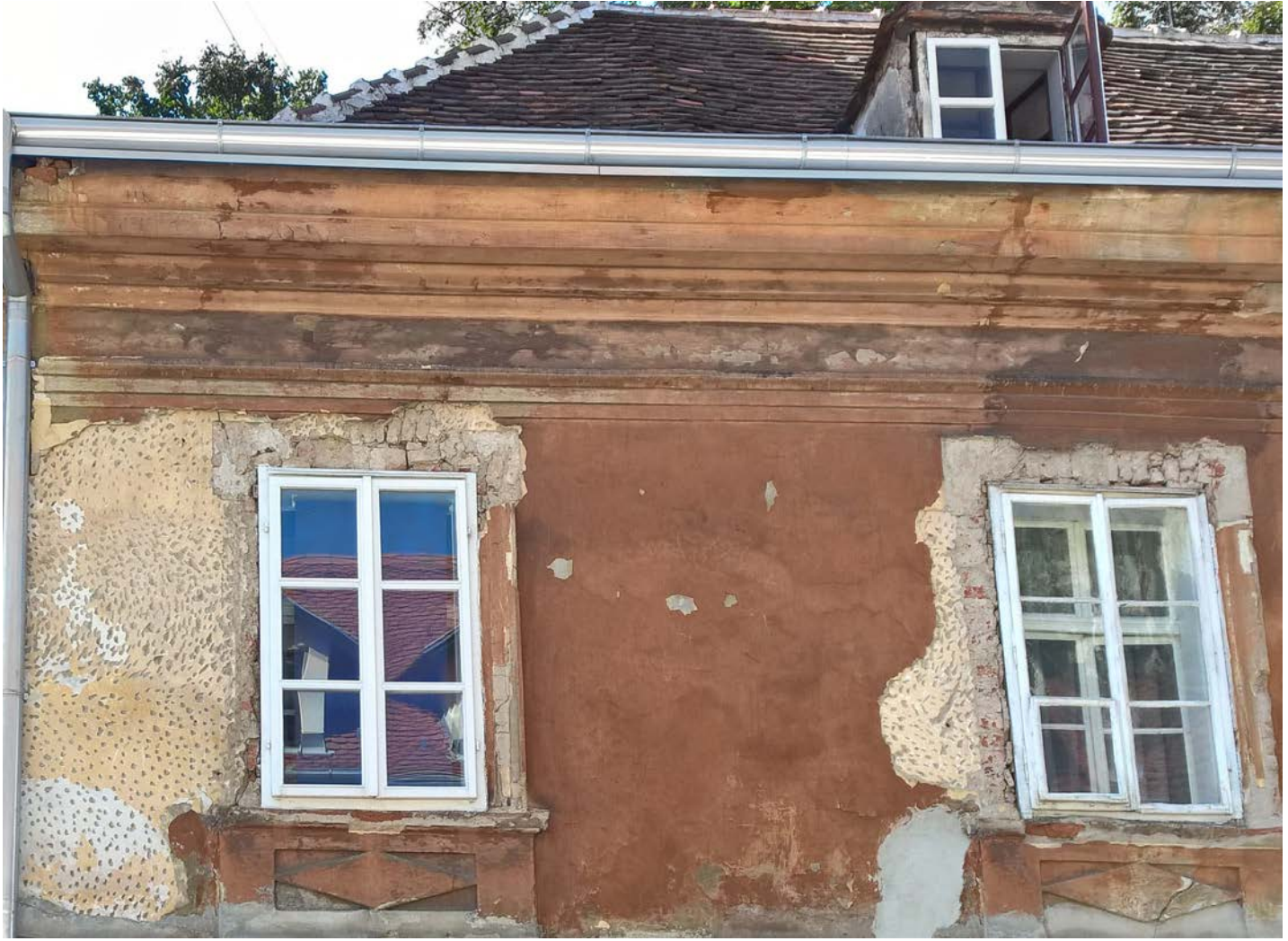
Losses of the top render layer allow a view of the layer beneath, showing traces of keying by hammering, historic building, Zagreb (Croatia); Photo: 2015, (Roland Lenz)
