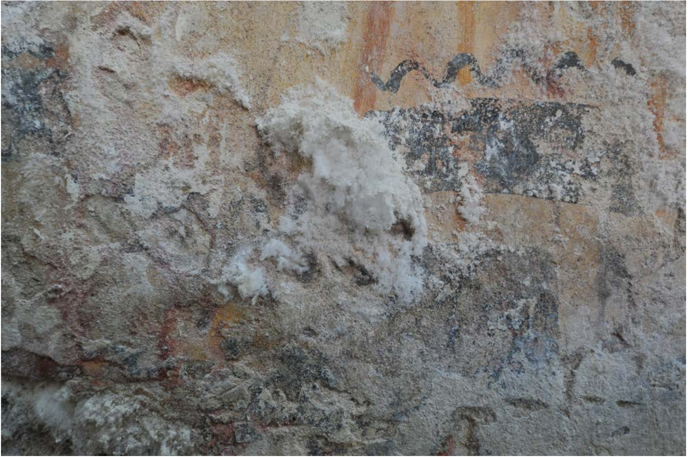
Salt crystals on the surface of a wall painting, no. 8 Universităţii Street, Cluj-Napoca (Romania), 2002; Photo: 2015, UAD (Adrian Rauca)
