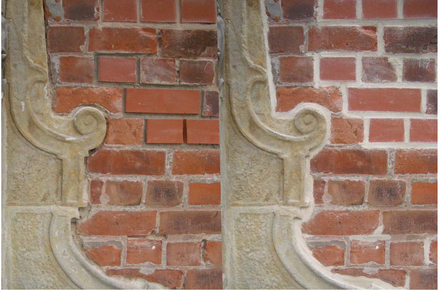
Raked (left) and repointed joints (right) of brick masonry and parts of a sandstone epitaph, Church of St. Gabriel, Haseldorf (Germany), end of 16th century; Photo: 2007 (Sophie Haake)
