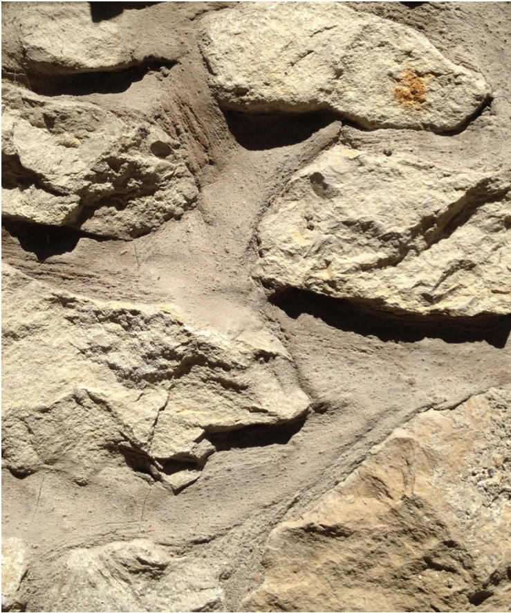
Natural stone masonry joint, Safranbolu (Turkey), 19th century; Photo: 2014, KBU (Aysun Özköse); Illustration: 2015, Raimar Heber based on a drawing by Oana Gui
