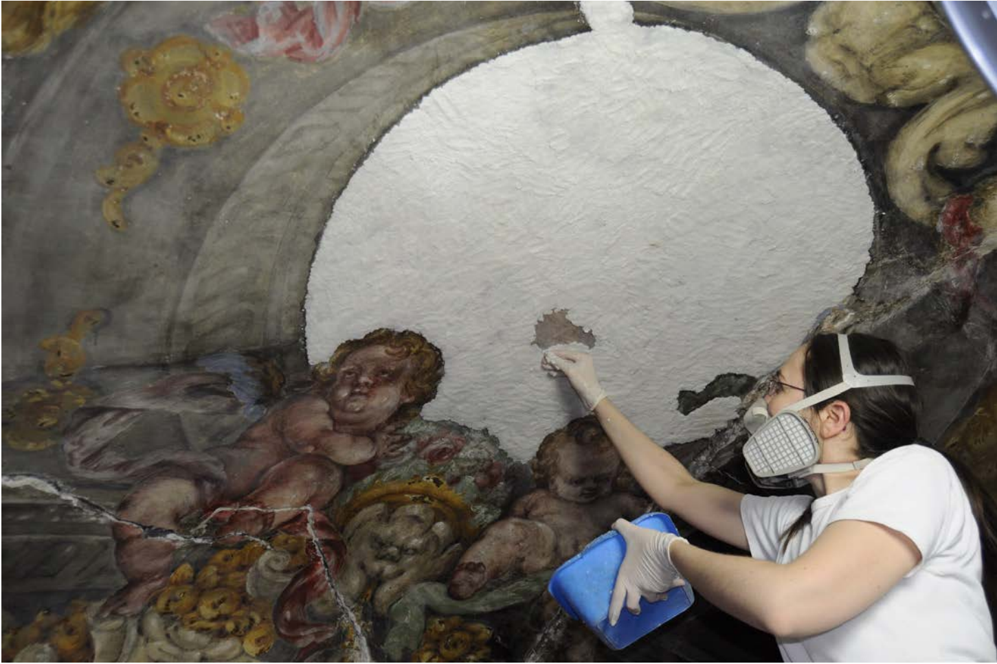
Application of a poultice, wall painting by Dionis Vidal, Church of San Nicolas Obispo San Pedro Martir, Valencia (Spain), 1694-1700; Photo: 2014, UPV
